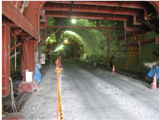
Figure 9: Tunnel where the specimen was cast
