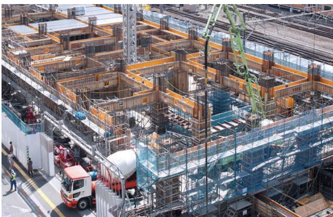
Figure 1. Showing construction site in Japan
