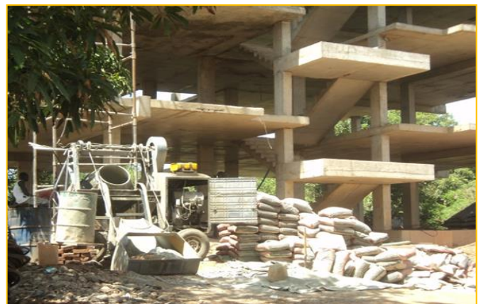
Figure 2. Showing construction site in South Sudan
